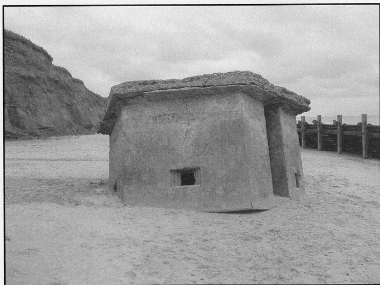
This upside-down pillbox on Happisburgh beach was one of hundreds built to defend the coast during the Second World War. It fell onto the beach in the 1970s when the cliffs were eroded from beneath it and is a potent reminder of the threat to the historic environment posed by coastal erosion.
